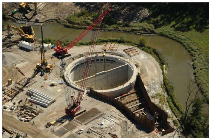
Figure 2-20: Caisson during construction
