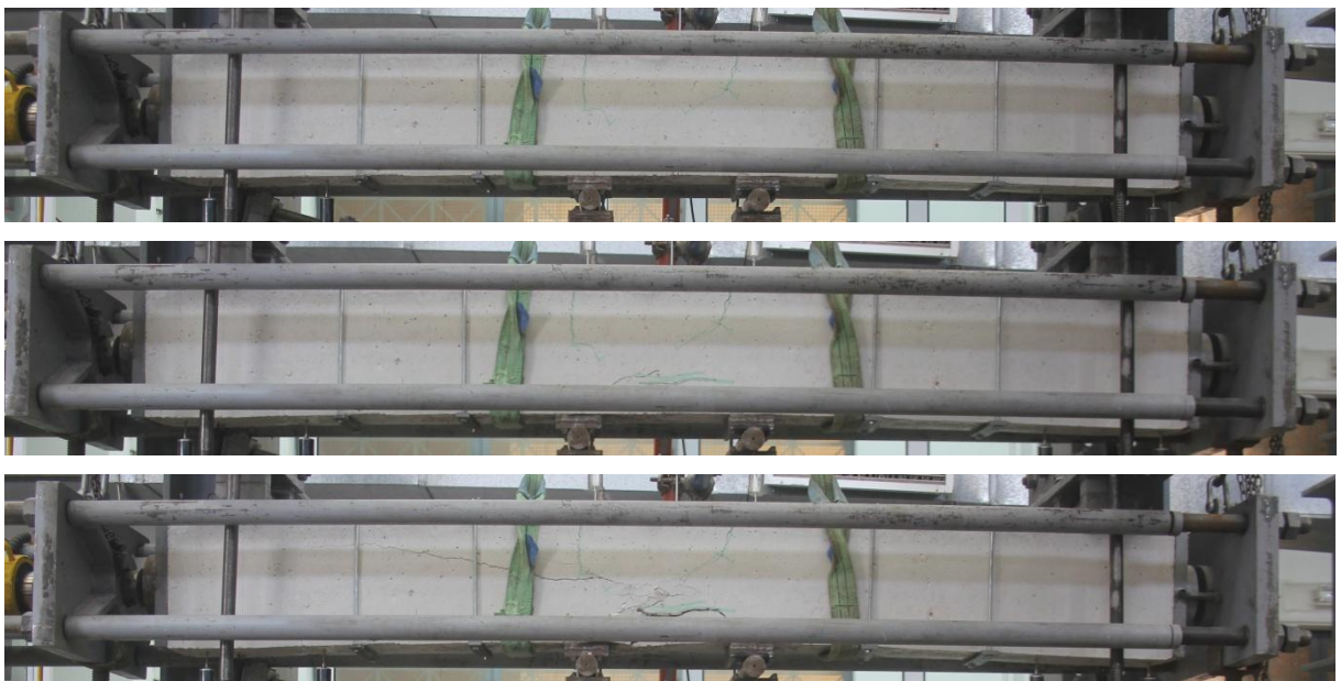
Figure 5.5: Crack pattern of the third beam.
