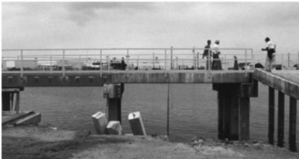
Waterfront structure, Port Hueneme, California
