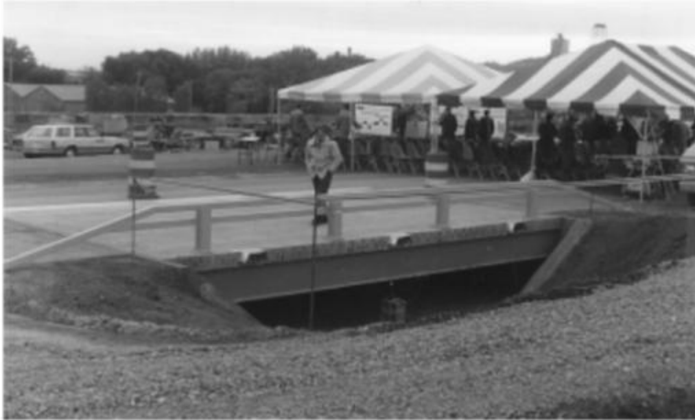
Composite prestressed bridge at Rapid City, South Dakota
