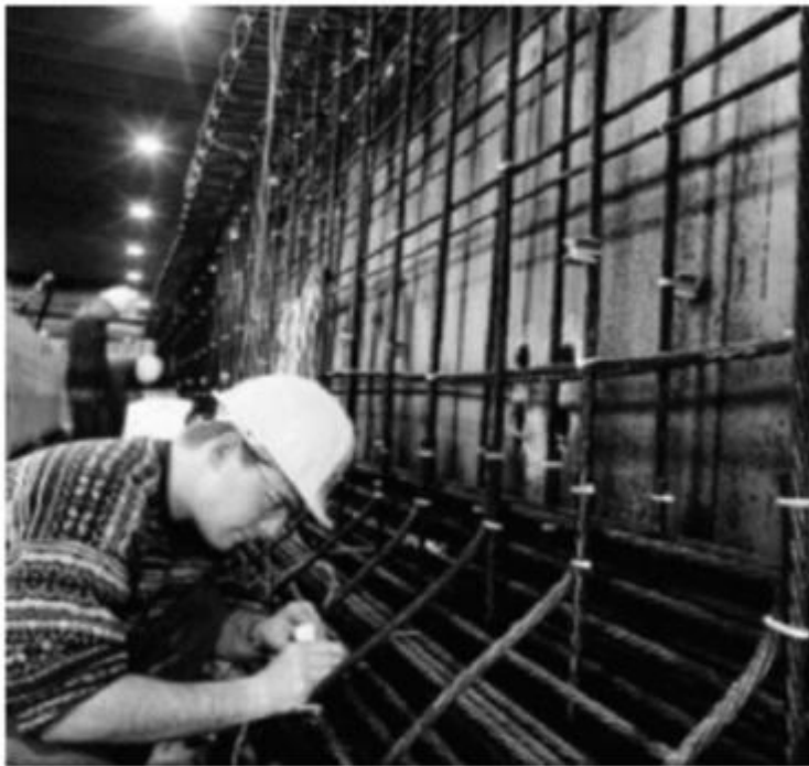
Installation process of the grating sensors on the girder surface
