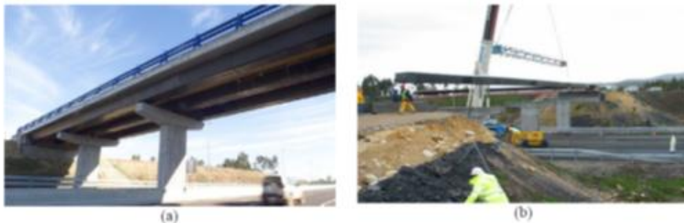
(a) View of the FRP girders of the Asturias bridge; (b) Positioning of one of the FRP girders during the construction phase.
