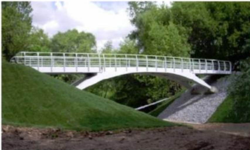
ApATeCh arched footbridge
