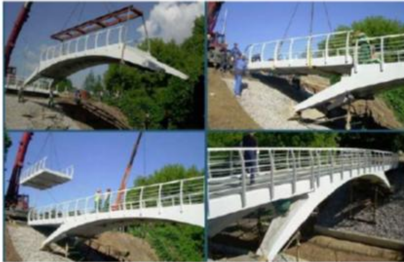
Installation of the footbridge
