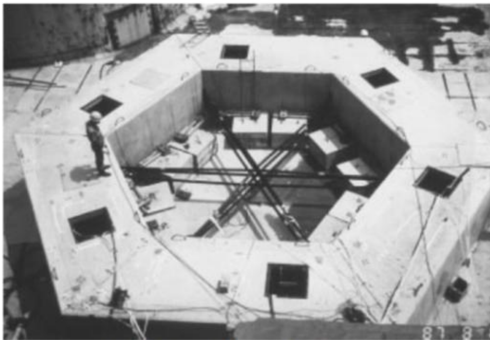
Hexagon marine structure, Kanagawa, Japan
