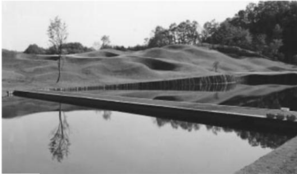
Floating bridge, Japan
