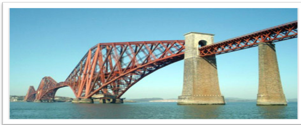
Σχ.1.17 Γέφυρα Firth of Forth
