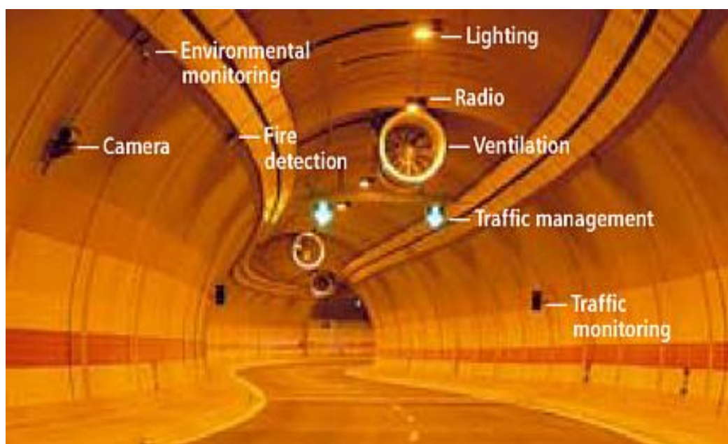
Figure 4: Technical aspects of a road tunnel system
