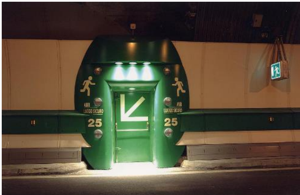
Figure 5: Emergency exits (PIARC 2007b)
